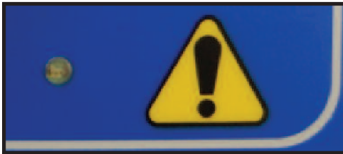
Figure 16.1.3-2: Warning light on the control panel at the operator's console
